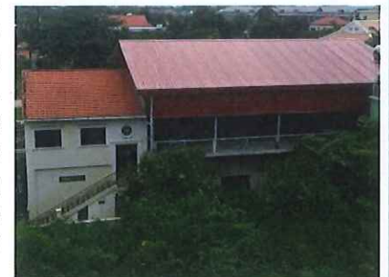
The exterior of our auditorium is nearly complete
